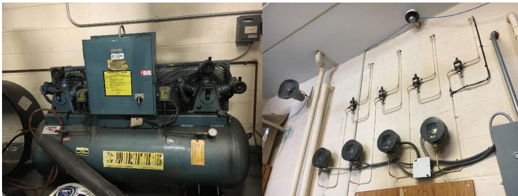
Figure 14 – Pneumatic Control System
