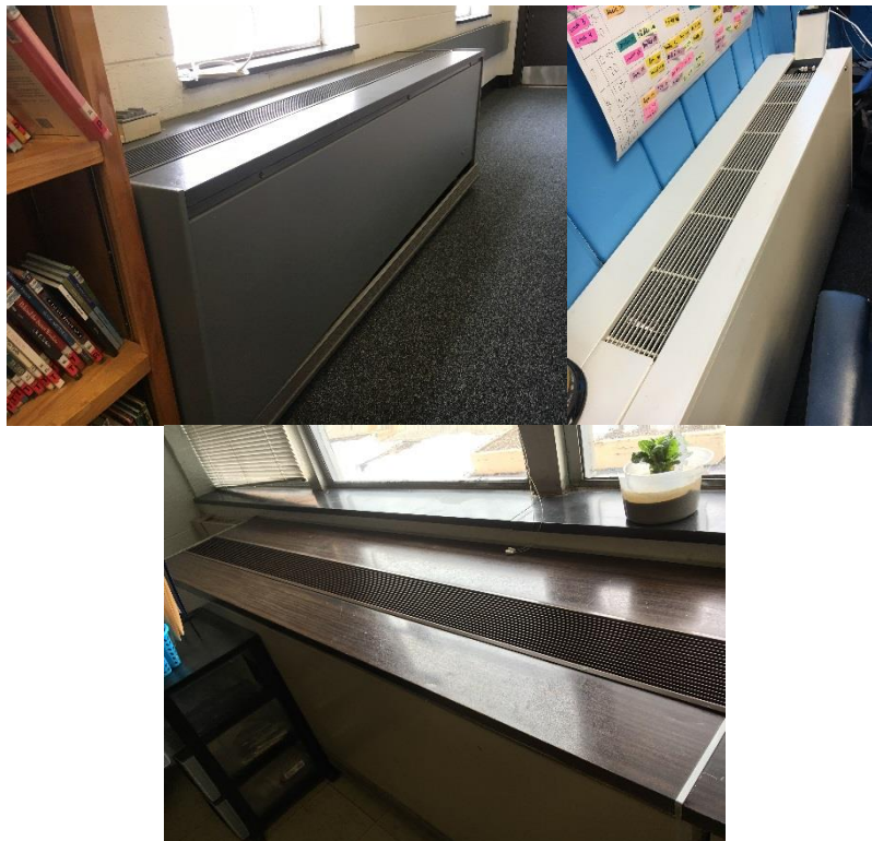
Figure 12 – Unit Ventilators
